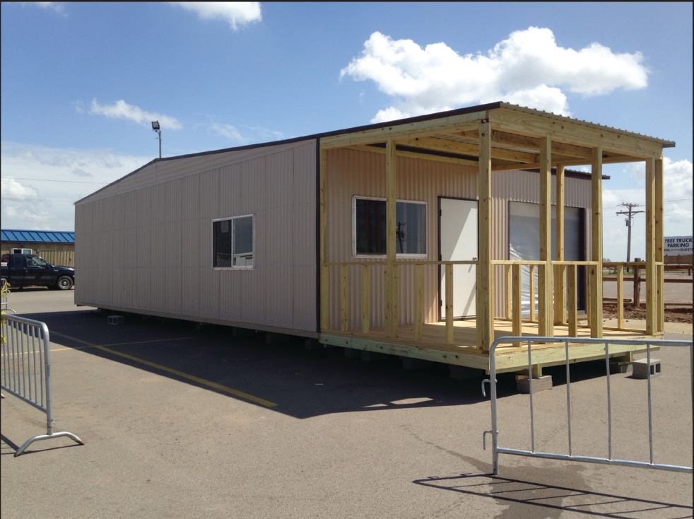
Construction progress on the Smoke Shop located by Sugar Creek Casino. More information in the President’s Report on page 2.
